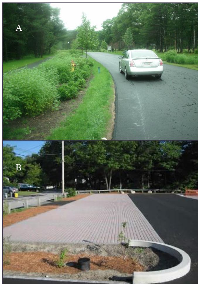
Figure 2. (A) Example of narrow residential road with a bio-swale, utilities, and single-sided sidewalk in Duxbury, MA. (B) Use of pervious pavers and bioretention practices in the landscape islands in spillover parking lot in Wilmington, MA.
