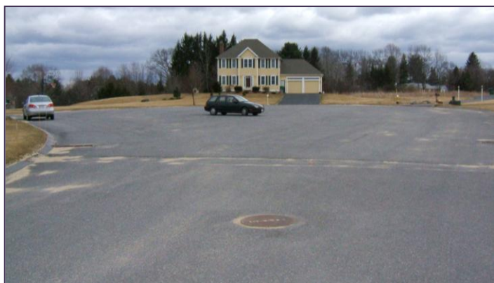
Figure 1. Unnecessarily wide cul-de-sacs and residential roads generate additional stormwater runoff, create un-friendly pedestrian environments, and increase overall construction costs.
